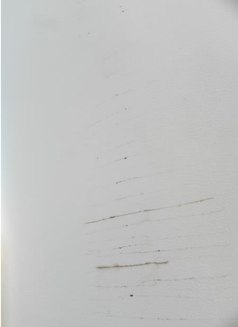
Figure 3. Parallel gel coat cracks.
